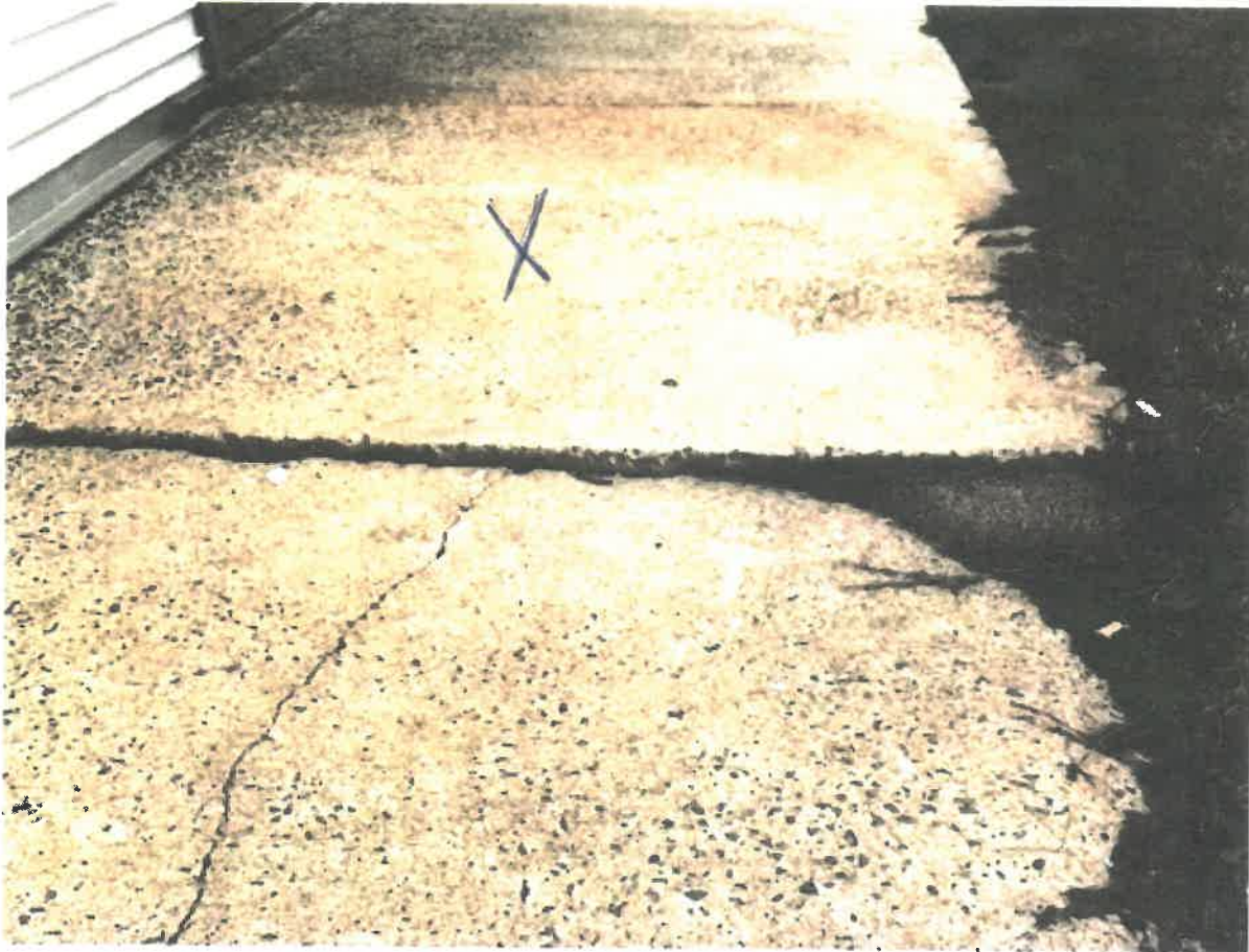
SIDEWALK AT REAR OF FACILITY IS UNEVEN. REPRESENTS A TRIP HAZARD.
