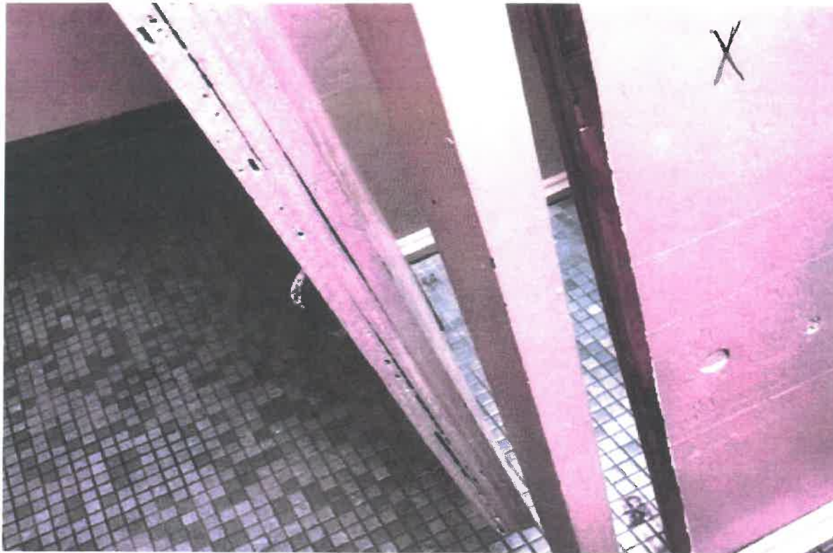
BATHROOM STALL DOOR MISSING LOCK AND THE FRAME IS DAMAGED.
